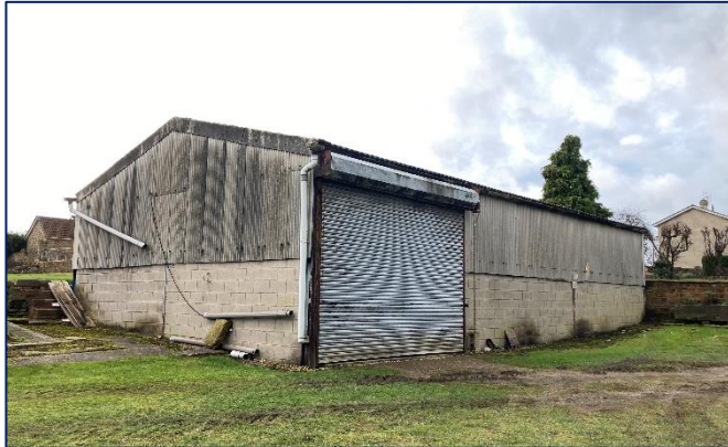
Agricultural Building to be demolished
