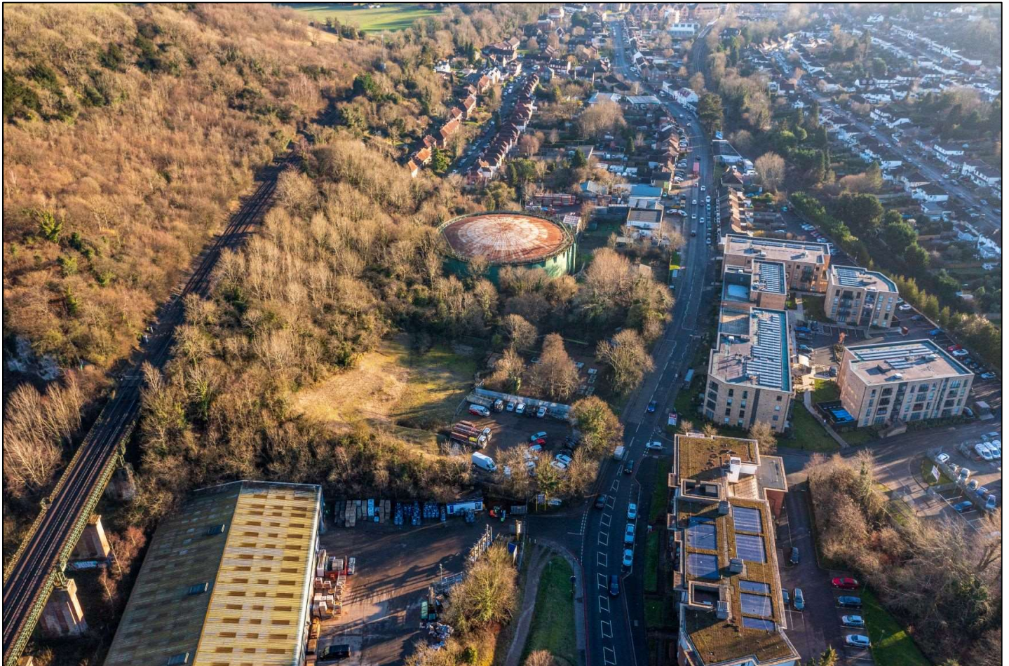
Aerial view of the Site looking south
