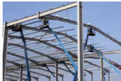
ALL STEELWORK IS PRE-FINISHED WITH A FACTORY APPLIED TWO PART EPOXY COATING
