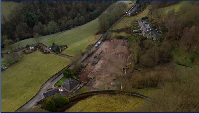
Main site looking west
