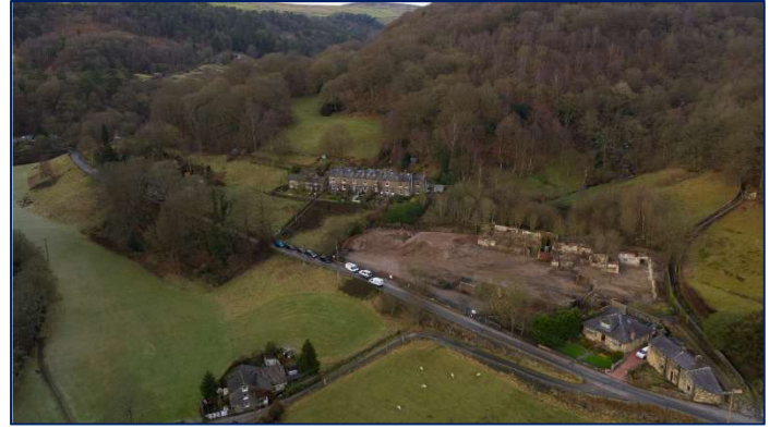
Main site looking west
